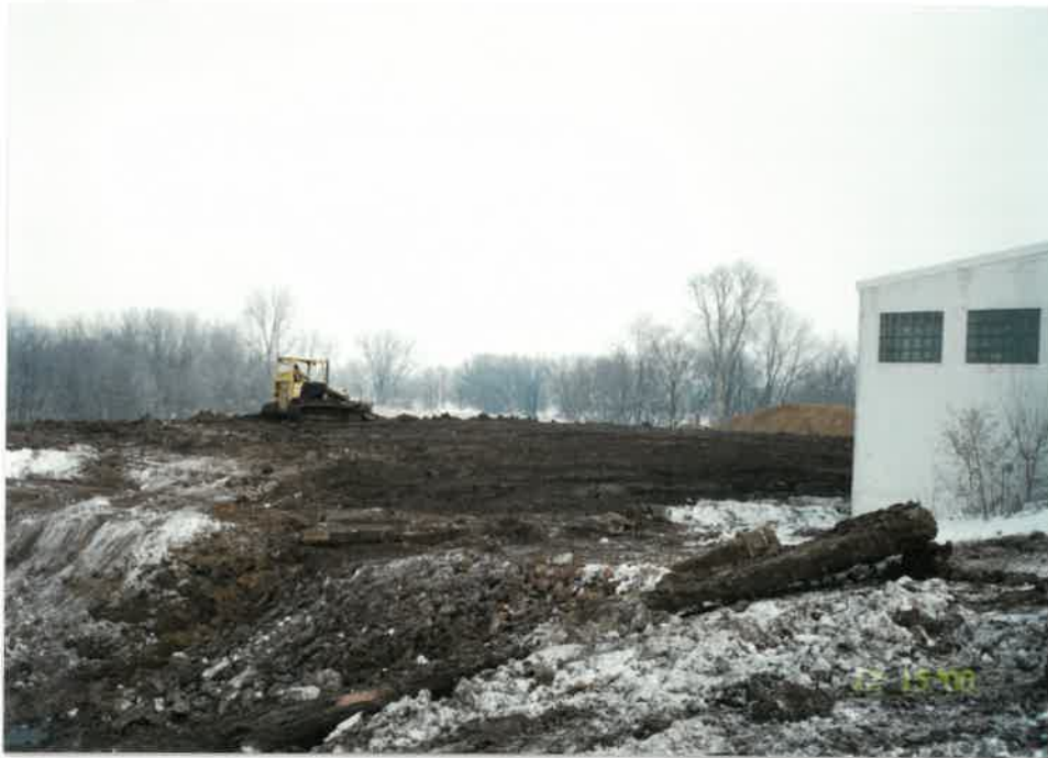
Photograph 3 December 15, 2000 Description: CAMU landfill top of sludge grades.
