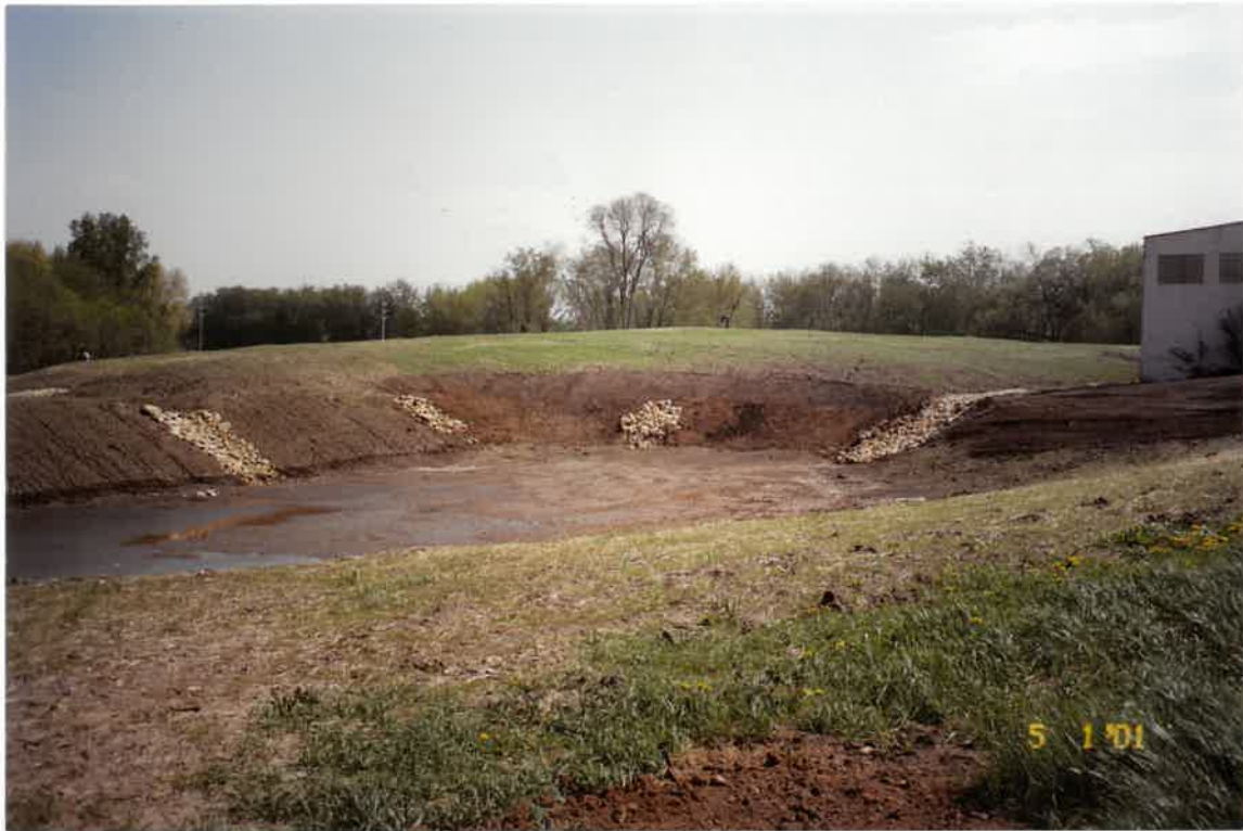
Photograph 13 May 1, 2001 Description: Sedimentation Basin No. 2 completed (Former location of Lagoon No. 1)
