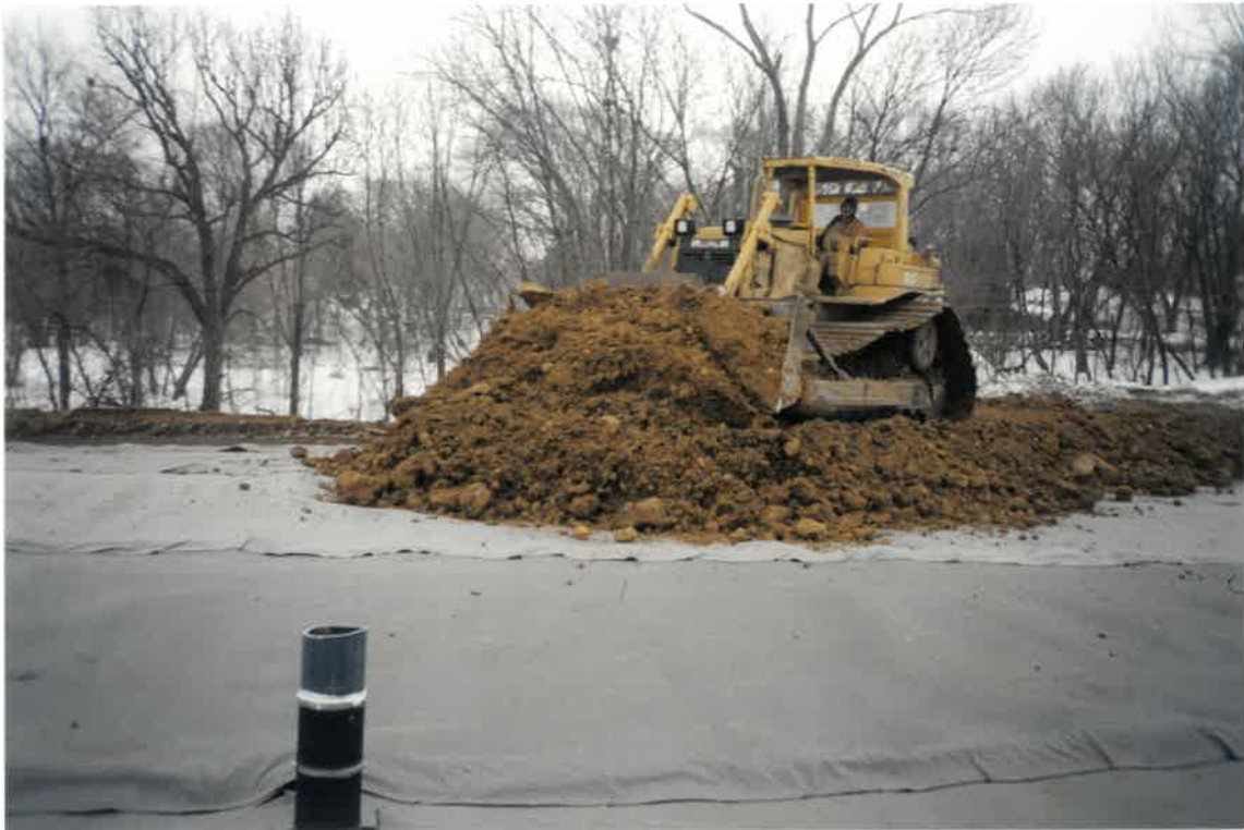
Photograph 9 January 19, 2001 Description: Placing rooting zone soils for CAMU landfill final cover.
