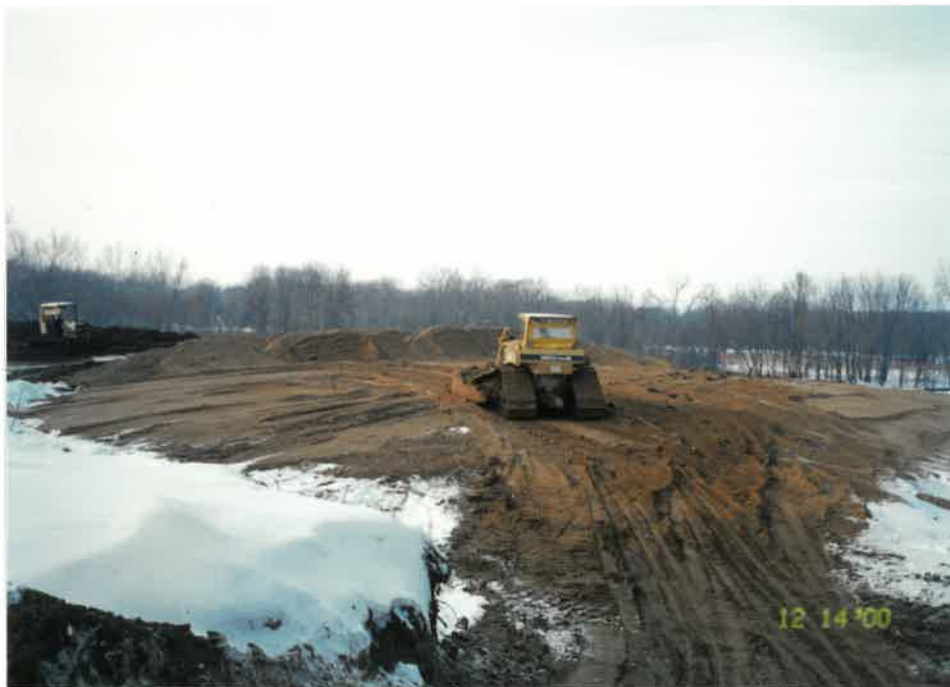
Photograph 2 December 14, 2000 Description: Placing grading/gas venting layer sand on CAMU.
