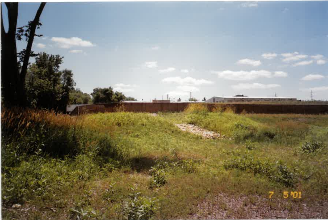
Photograph 17 July 5, 2001 Description: Security fencing around the CAMU looking south, riprapped spill way from Sedimentation Basin No. 1 in the foreground.
