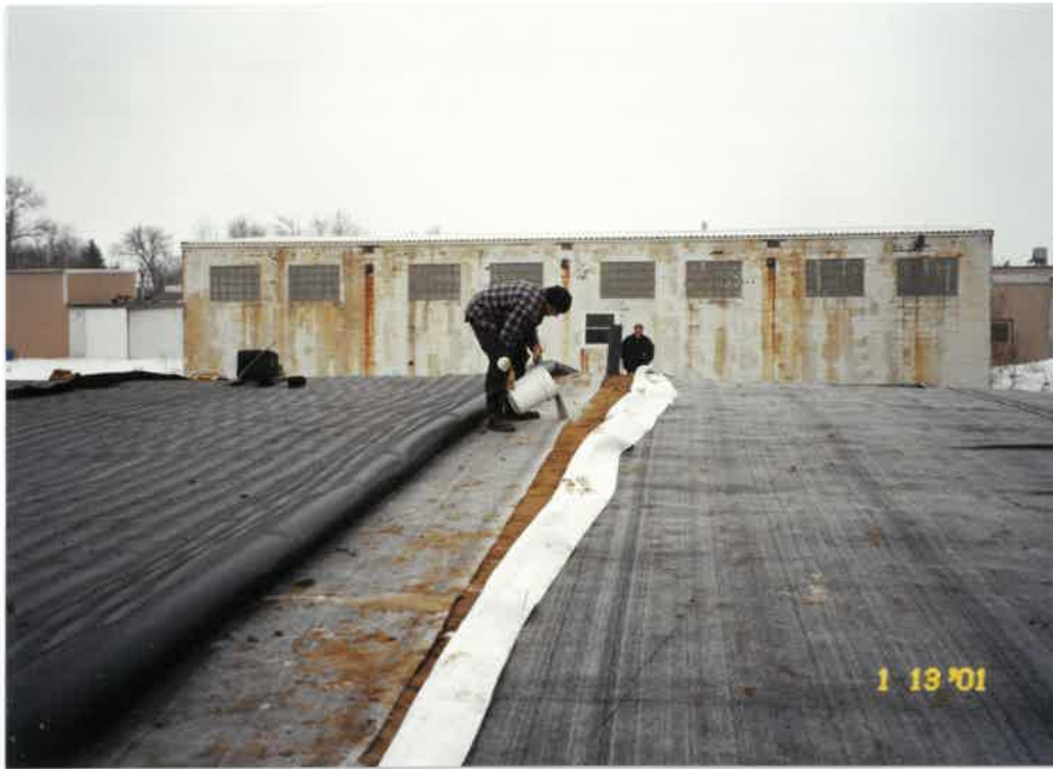
Photograph 7 January 13, 2001 Description: Placing GCL and geomembrane panels on CAMU landfill cap.
