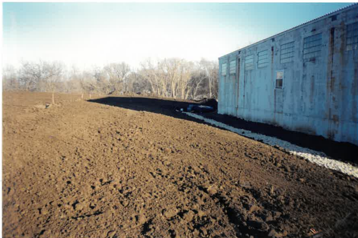
Photograph 10 January 25, 2001 Description: CAMU landfill final cover topsoil and rooting zone drainage system.
