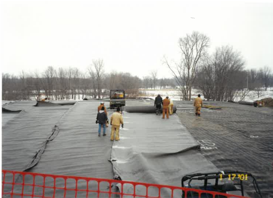
Photograph 8 January 17, 2001 Description: Deploying geocomposite on CAMU landfill cap.
