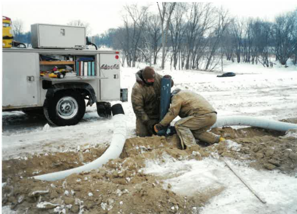
Photograph 4 December 26, 2000 Description: Installing gas vent piping in grading/gas venting layer.
